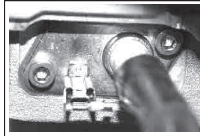
Ignition / Ionisation Electrode
